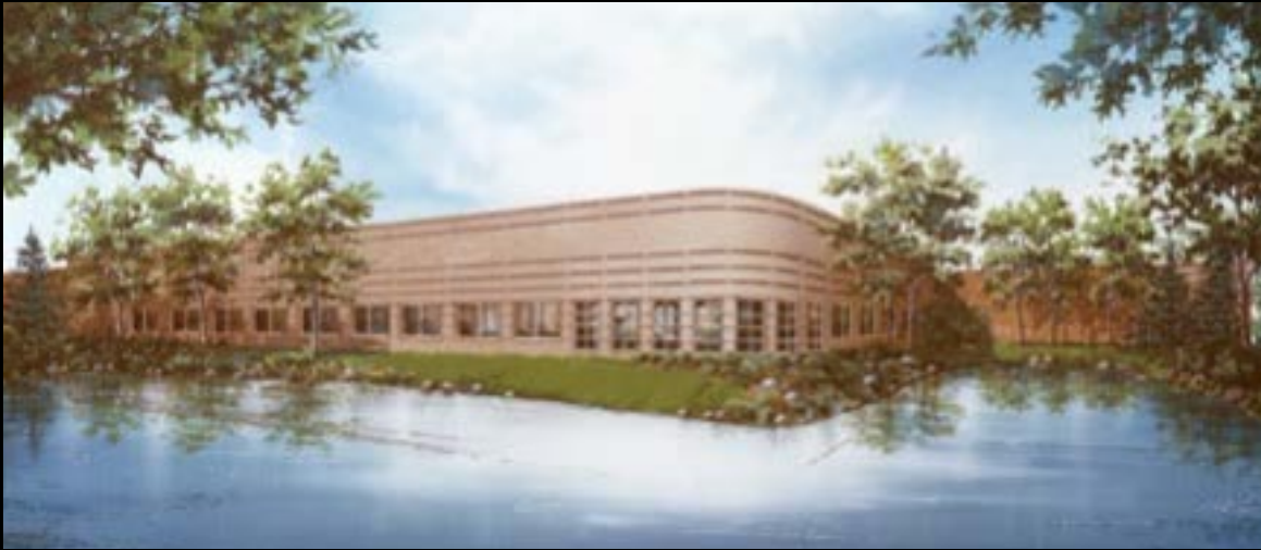
Vernon Hills, Illinois: Headquarters/Plant
